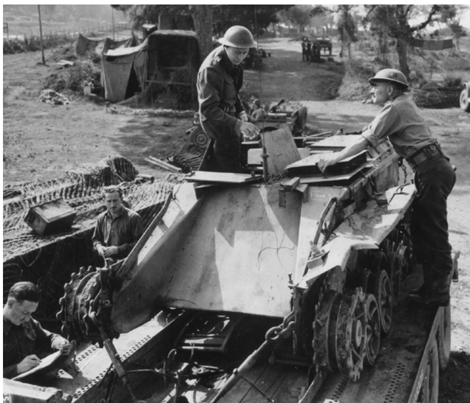
A Borgward B IV from PzAbt (Fk) 301 captured by British troops near Nettuno, Italy, is loaded on a transport vehicle to be taken away for evaluation. The tracks are badly damaged due, probably, to the vehicle being guided in to clear a minefield. The bay for the 450kg explosive charge is empty. (NARA)
